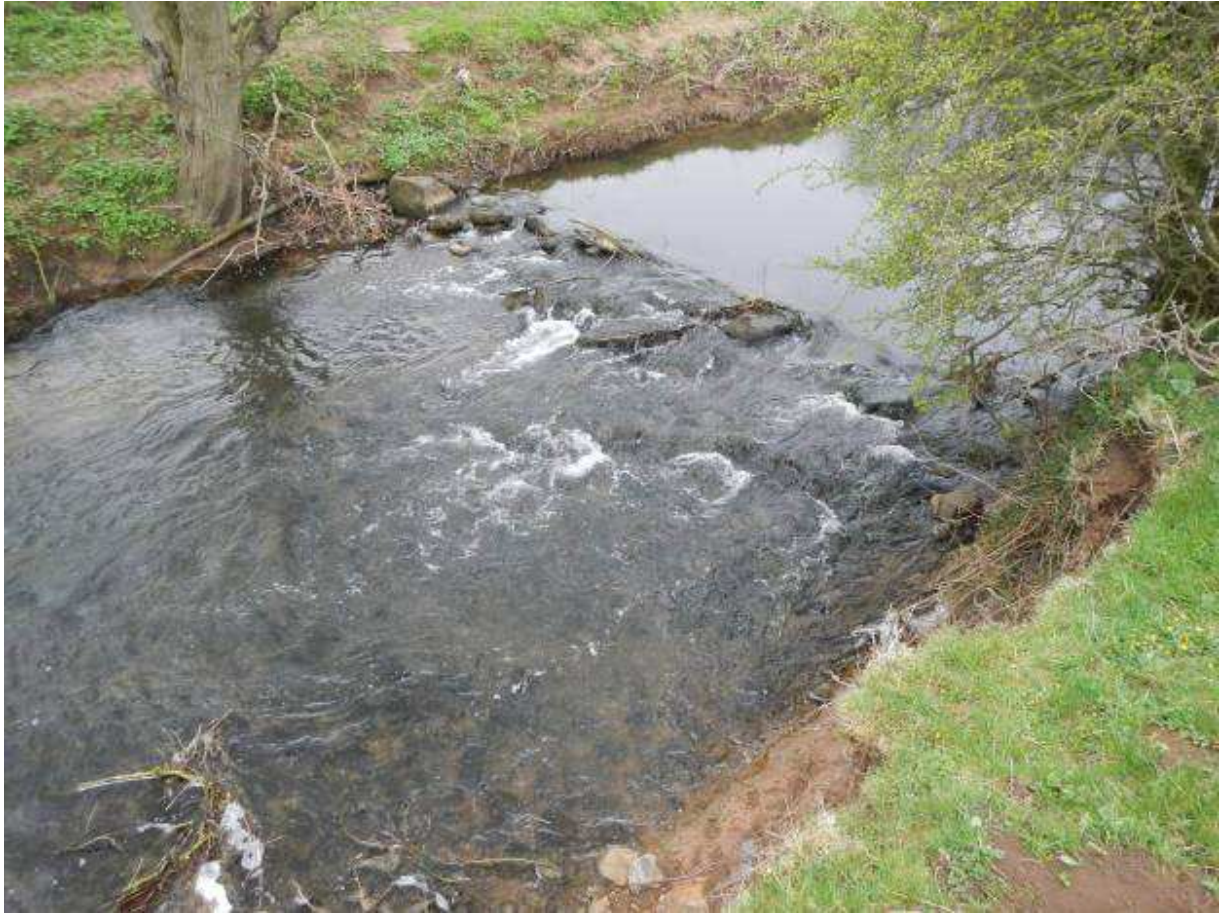
Figure 13. Small weir downstream of the A168 (NGR - SE4367880518). Removal of 400-500mm of width in the central area down to bed level, on this and other similar weirs would be very beneficial.
