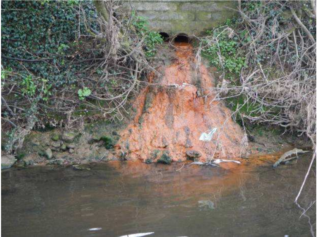
Figure 11. Metalliferous (probably hydrated iron oxides) discharge assumed to be from an old gravel working (NGR - SE4360780276).
