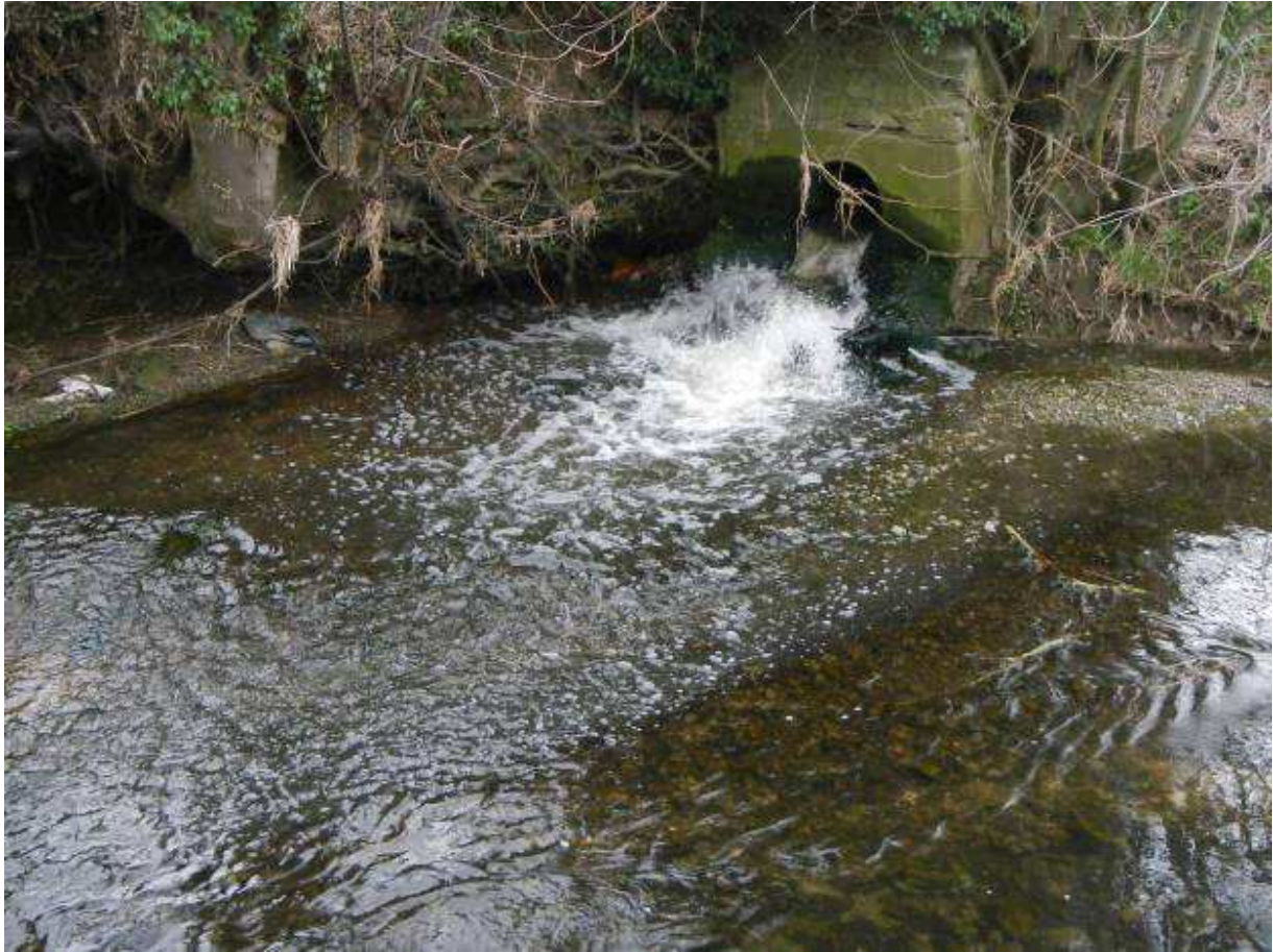
Figure 12. Grey water discharge from the sewage works (possibly elevated in nitrates and phosphates, however, little evidence of detergent contamination). This should be reported to the EA as a possible chronic pollution (NGR - SE4361180294).
