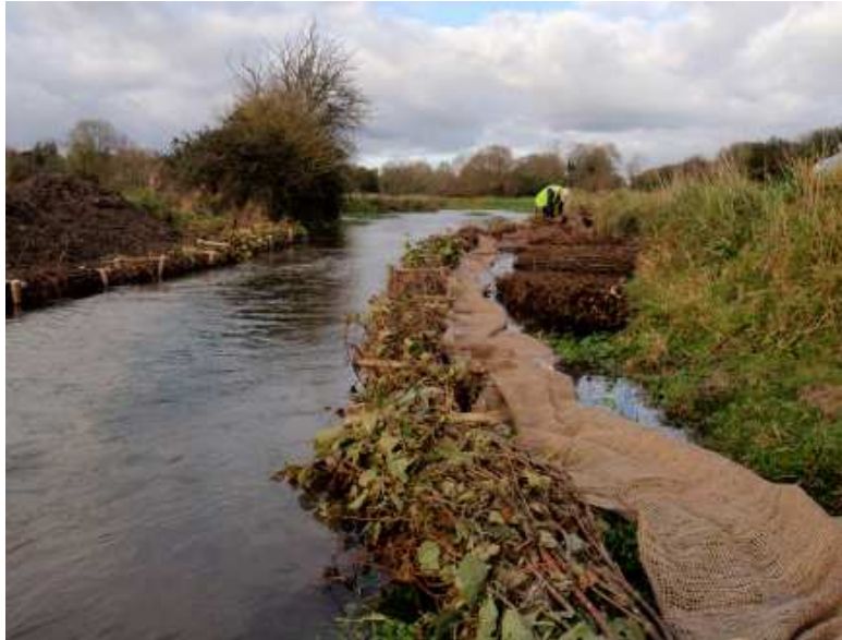
Figure 14. Bank creation using willow faggots and brush backfill. This example also includes the use of hessian or coir.
