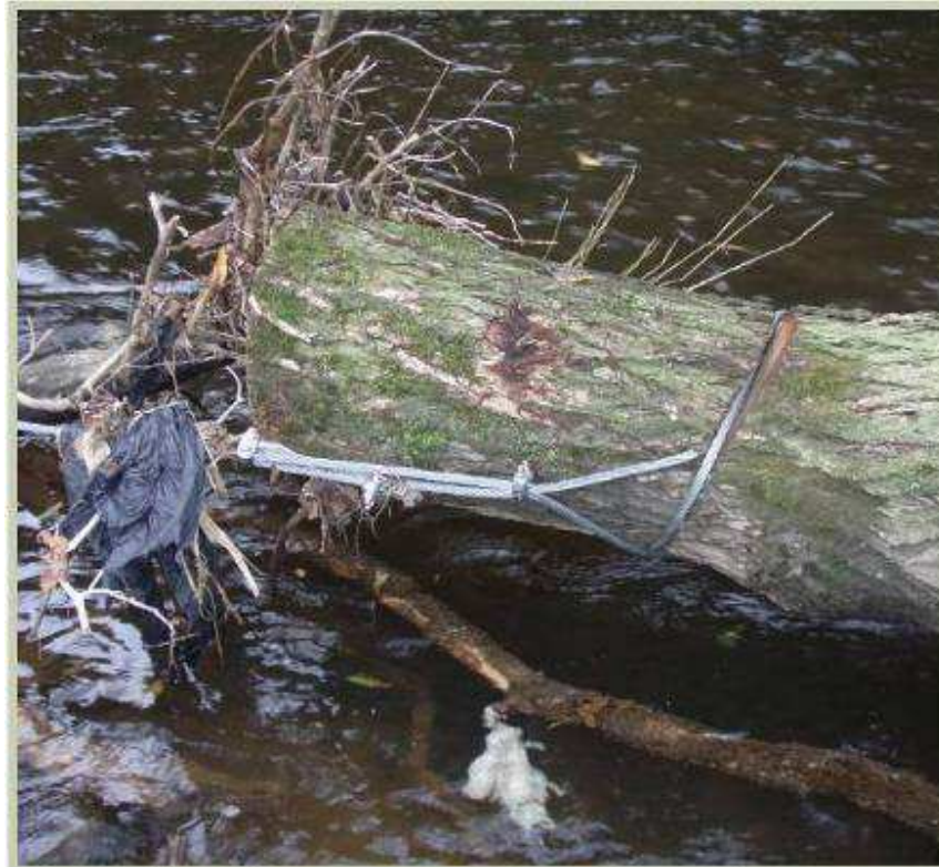
Figure 17. Cabling for a tree kicker.
