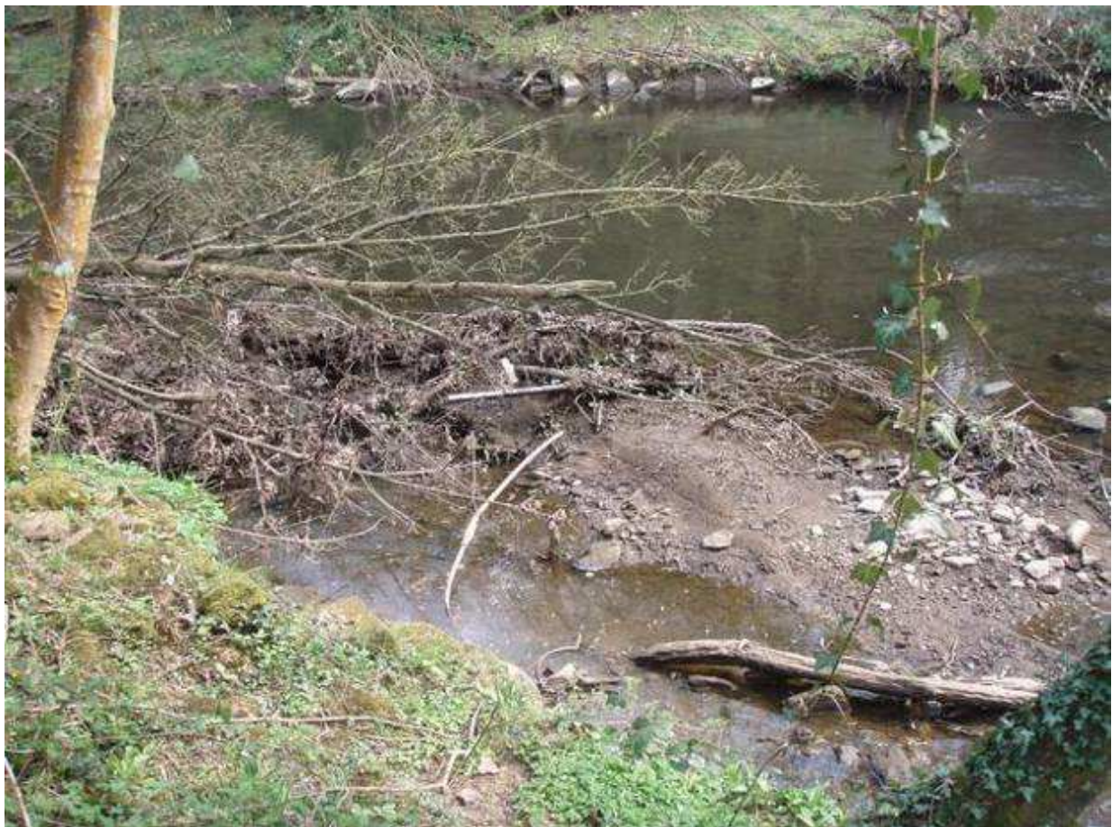
Figure 16. Note the narrowing effect through significant gravel and sediment accumulation (centre and right of shot) in the sheltered area downstream of the tree kicker.
